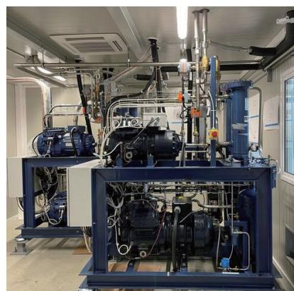
Fig. 3 System A room two modules installed side by side.
