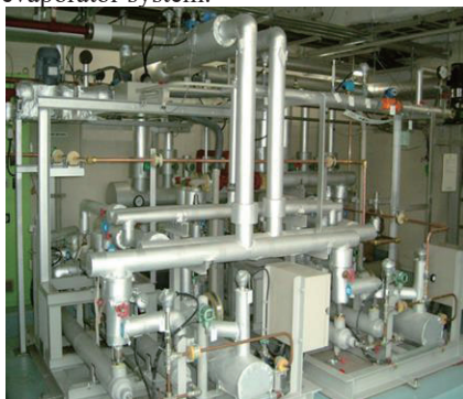
Fig.2 CO 2 Heat Pump System
